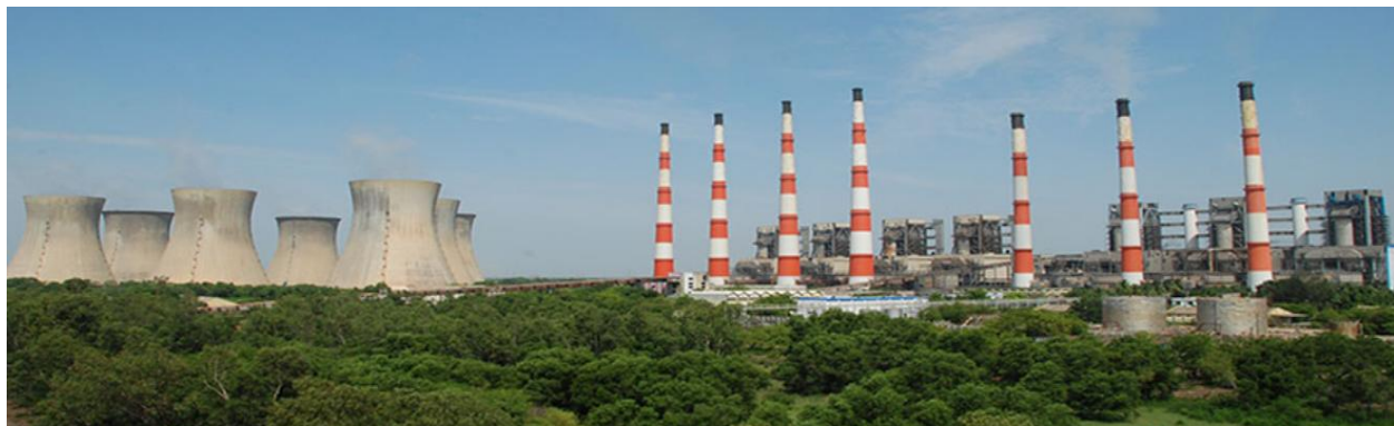
Over View of Thermal Power Station-II, NLC, Neyveli
